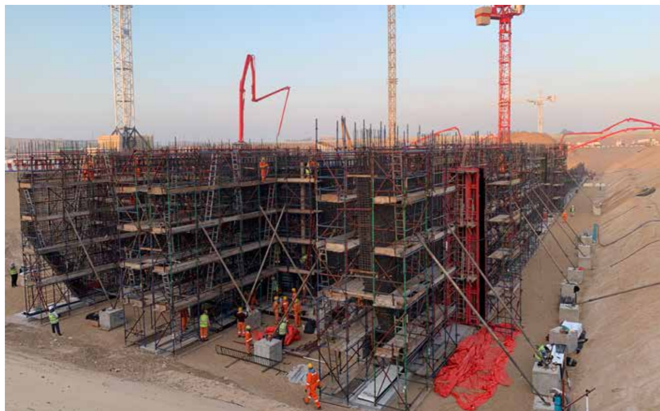
SITE OF THE FUTURE DUBAI WASTE-TO-ENERGY PLANT, UAE
