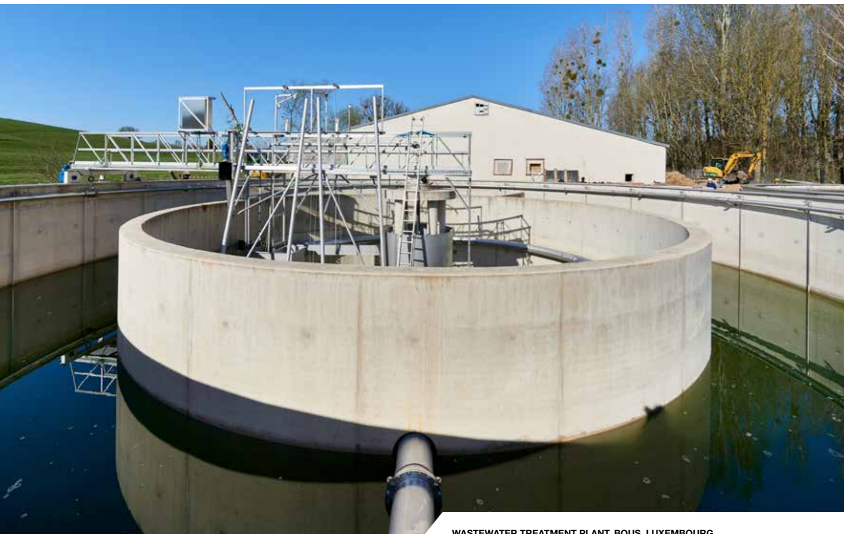
WASTEWATER TREATMENT PLANT, BOUS, LUXEMBOURG
