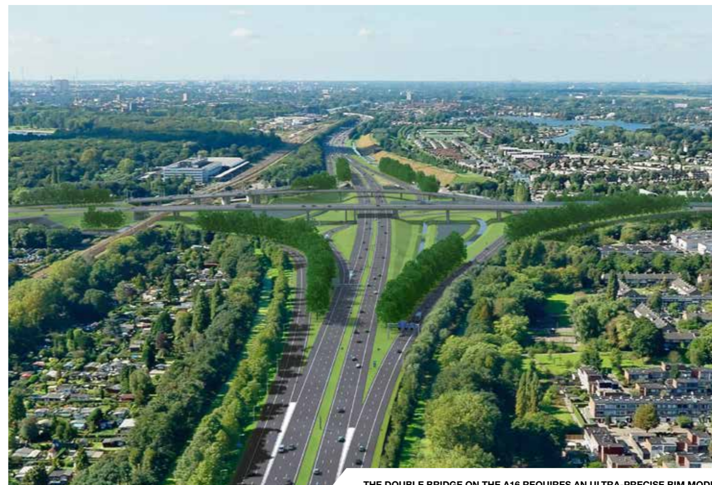
THE DOUBLE BRIDGE ON THE A16 REQUIRES AN ULTRA-PRECISE BIM MODEL
