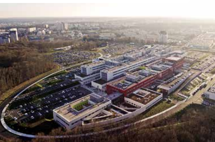
HOSPITAL GROUP SUD ILE DE FRANCE, MELUN, FRANCE
